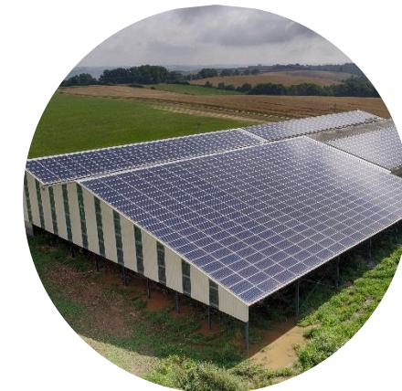
Hangar agricole Tarn (81)
