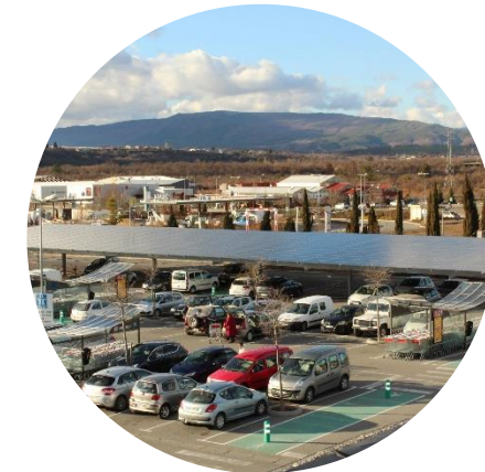
Ombrière Parking centre commercial
